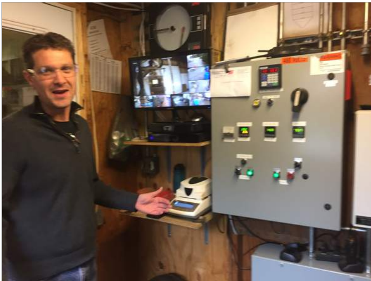
Plant manager Bill Peebles of Palermo gives a tour of the control room. (Photo by: Jordan Bailey)
